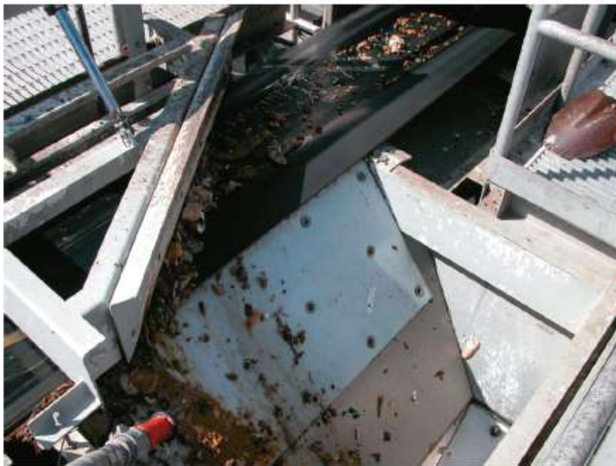
FIGURE 25.5 Removal of small debris via a “moving screen.”
