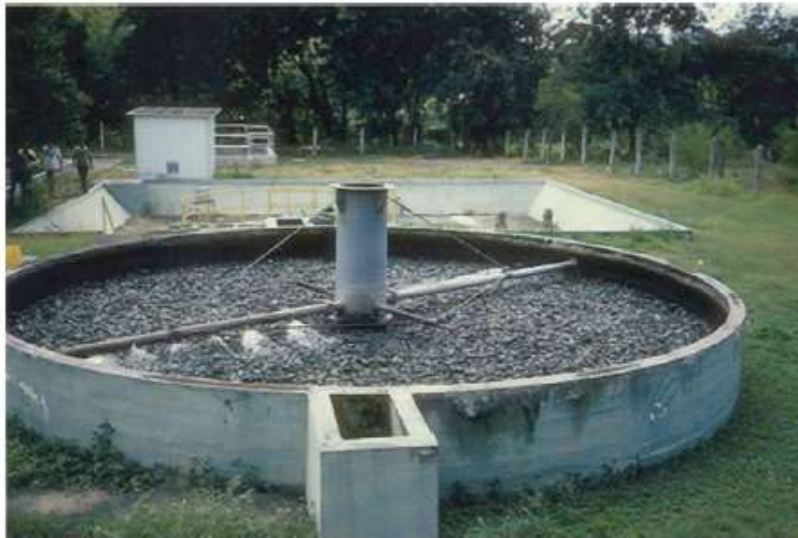
FIGURE 25.7 A trickling filter bed. Here, rocks provide a matrix supporting the growth of a microbial biofilm that actively degrades the organic material in the wastewater under aerobic conditions.
