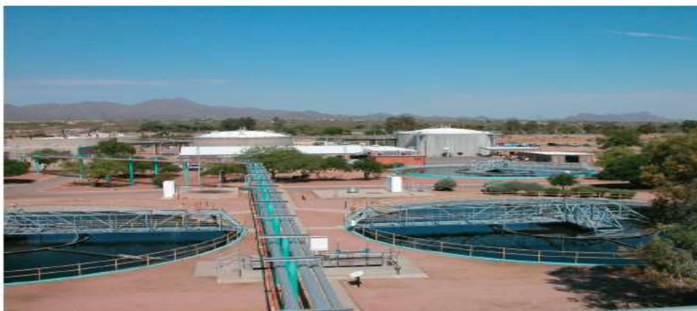
FIGURE 25.6 Three clarifiers (foreground—blue) where suspended organic solids settle out as primary sludge. Also see the two anaerobic sludge digestors in the background (white).
