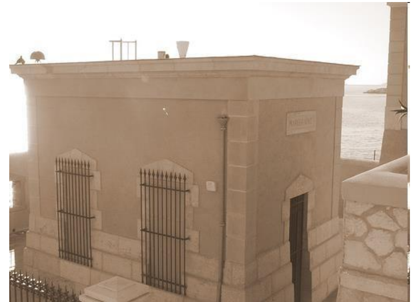
Tide gauge of Marseille, where '0' topography is defined in France
